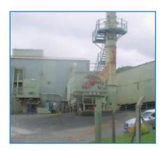
solution started with a 110kW ABB standard drive. "The fan had its damper placed in the fully open position and dryer pressure was then controlled via a pressure transmitter feeding back to the drive." he explains.
